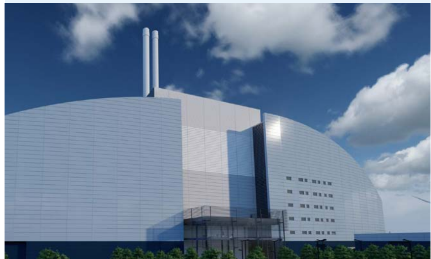
A render of the Skelton Grange facility under construction
